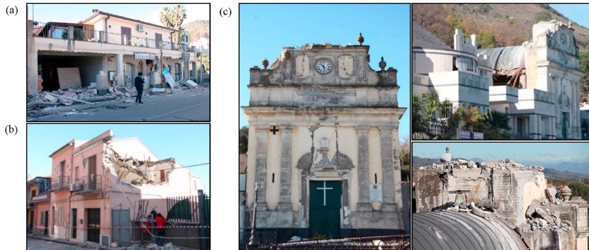
Fig. 2. Damage caused by the 26 December 2018 earthquake in Fleri (Zafferana Etnea): (a) Breakage of partitions in reinforced concrete buildings; (b) Partial collapse of a masonry building; and (c) Details of the damage to the facade of the church in Fleri restored after the 1984 earthquake.
