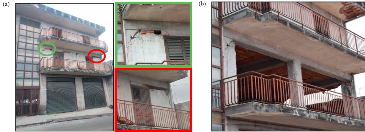
Fig. 7. Structural damage in the investigated building due to the 26 December 2018 earthquake: (a) Shear failure of the column (green shape) and breakage of infill panels (red shape), and (b) Subsequent demolition of infill panels.
