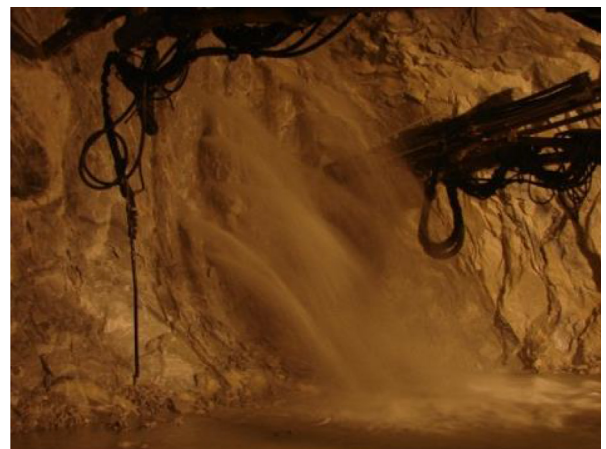
Fig. 3. Water inrush in a deep hard rock tunnel.
