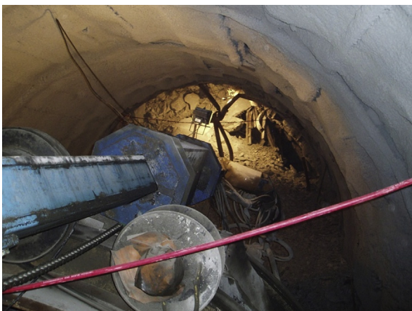
Fig. 7. “11.28” extremely intense rockburst in the drainage tunnel in Jinping II hydropower station.
