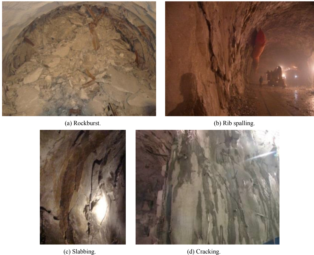
Fig. 2. Typical rock failures under high stress conditions.
