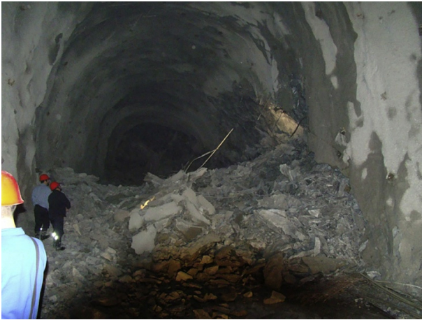
Fig. 6. Extremely intensive rockburst in auxiliary tunnel B in Jinping II hydropower station.
