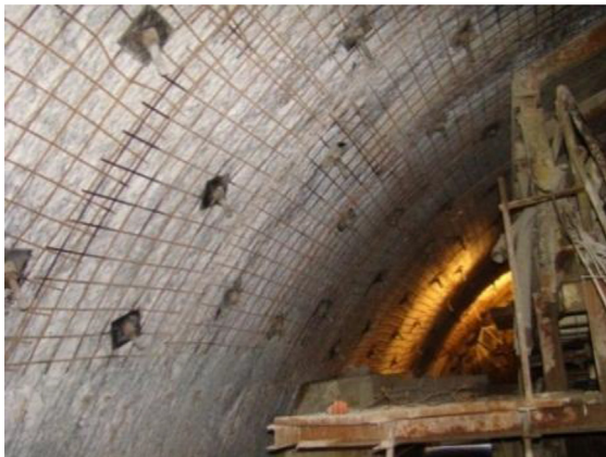
Fig. 30. On-site support effect of rockbolts with parameters designed by proposed method in Fig. 28.
