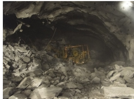
Fig. 27. Failure state of surrounding rocks at section k9 + 810 in headrace tunnel #4.
