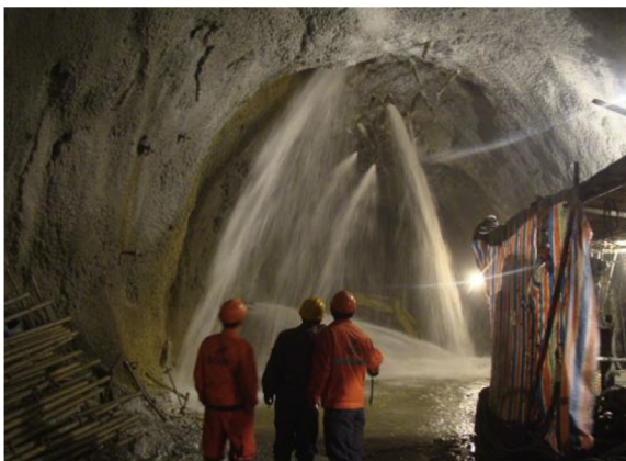
Fig. 23. An example of high-pressure and large-volume groundwater infiltration during tunnel excavation.
