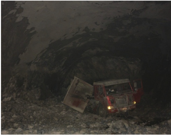
Fig. 16. An example of strong rockburst in a deep tunnel of the Jinping II project.
