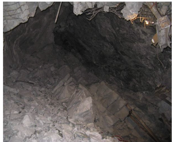
Fig. 18. An example of tectonic burst in a deep tunnel of the Jinping II project.
