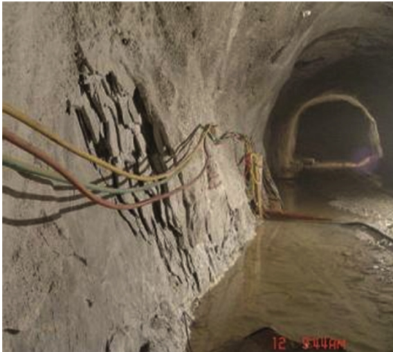
Fig. 13. An example of fracture-induced damage to the surrounding rocks in a deep tunnel of the Jinping II project.
