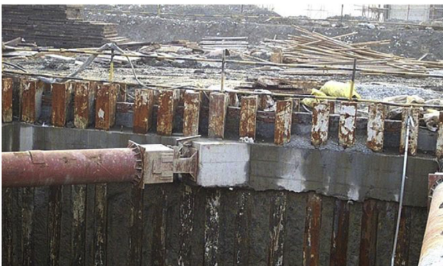
Fig. 3. Photo of a constructed DSMW in Tianjin subway project.
