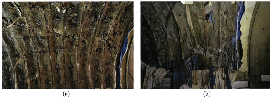
Fig. 15. Damage condition of steel support: (a) Right side of span S166, and (b) Left side of span S167.
