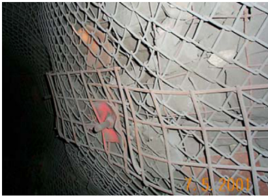
Fig. 15. Rockburst support system comprising strong meshes, mesh straps, and energy-absorbing yield rockbolts in a Canadian deep mine (photo by B. Simser).
