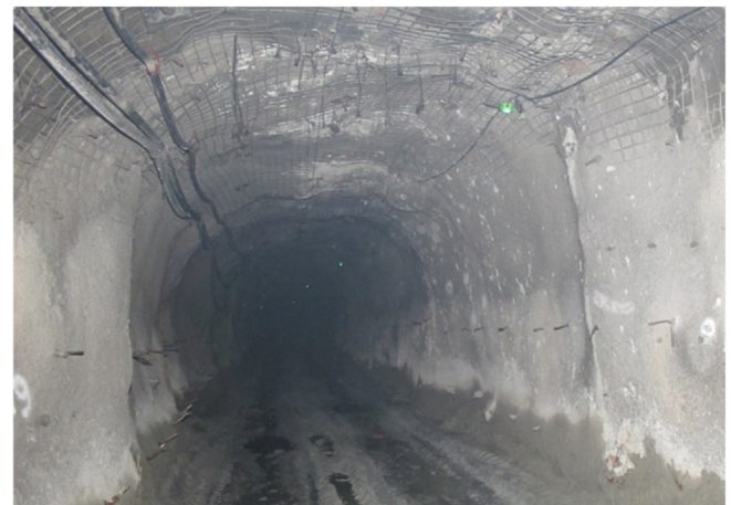
Fig. 9. Drill drive in DMLZ after a local magnitude M = 2 event in close proximity. Note that there is minimal wall damage and little shotcrete ejection despite signs of floor heave (Photo: Courtesy PT Freeport Indonesia).
